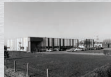
Plant of Le Coudray St Germer (France)
